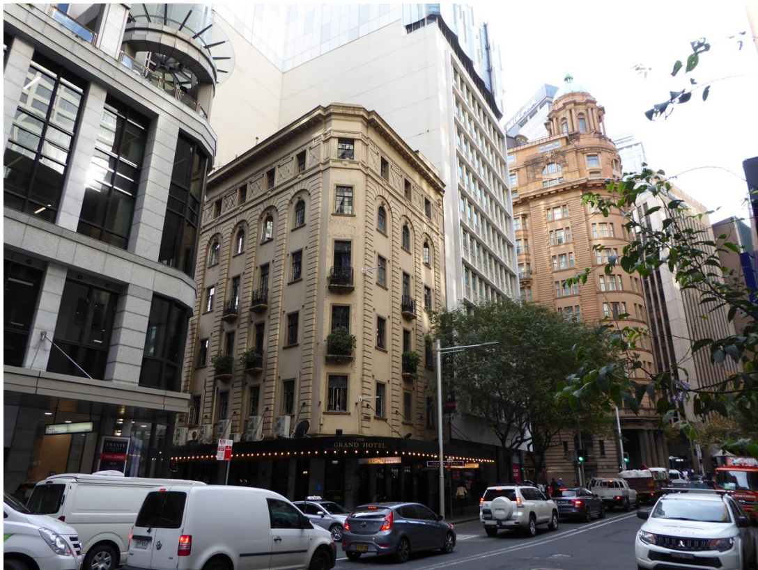
Figure 5. Northern side of Pitt Street, opposite the subject site
