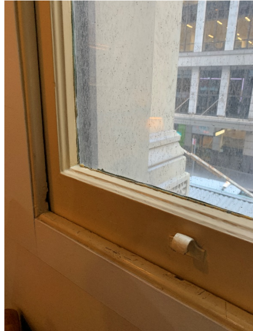
26 Detail view of surviving window architrave and internal features
