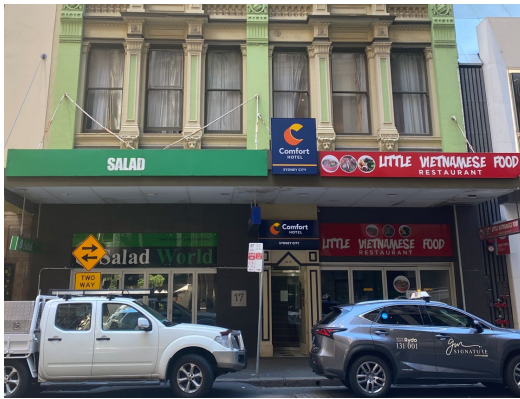
15 View of ground floor tenancies. Note lion heads, just above awning. Source: TKD Architects, 2021
